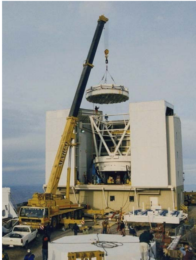
Figure 2. The \phi 6.5 m mirror is lowered into its cell March 25, 1999. Photo courtesy of Marco Crane.
