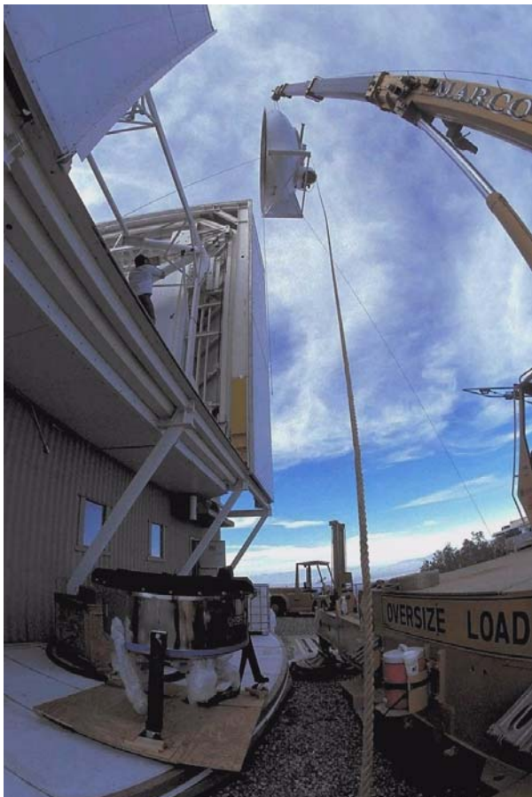
Figure 15. The vacuum head is lifted over the telescope structure (left) and lowered into place (right).
