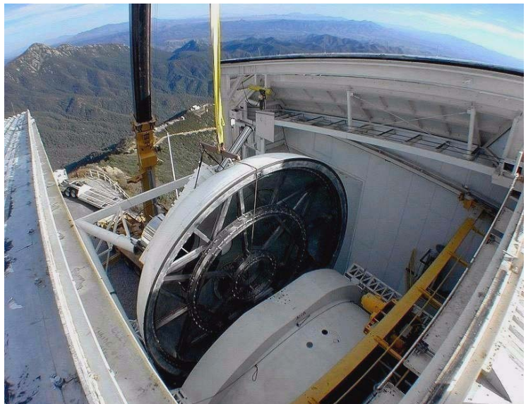
Figure 15. The vacuum head is lifted over the telescope structure (left) and lowered into place (right).
