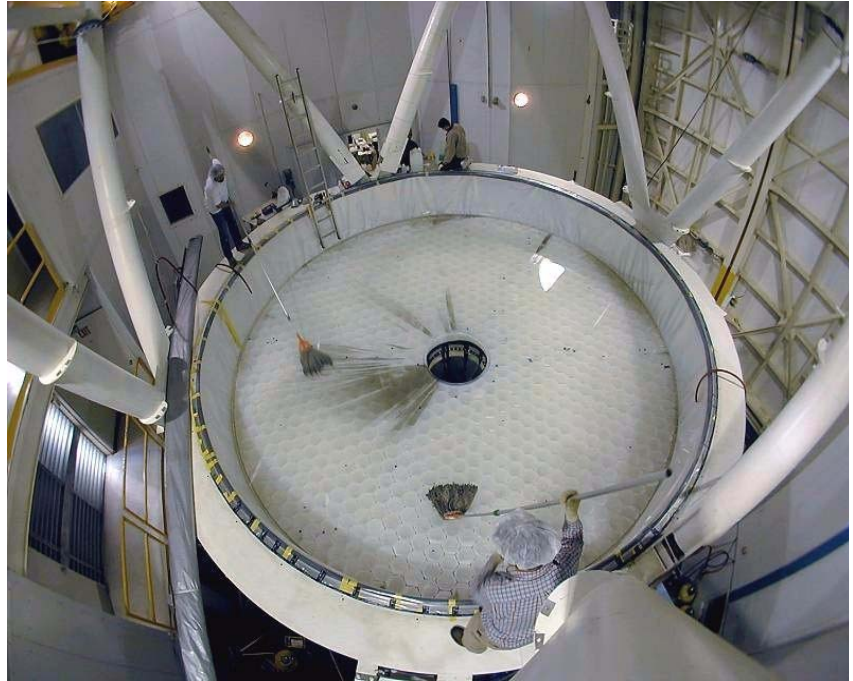
Figure 12. The old aluminum is removed.
