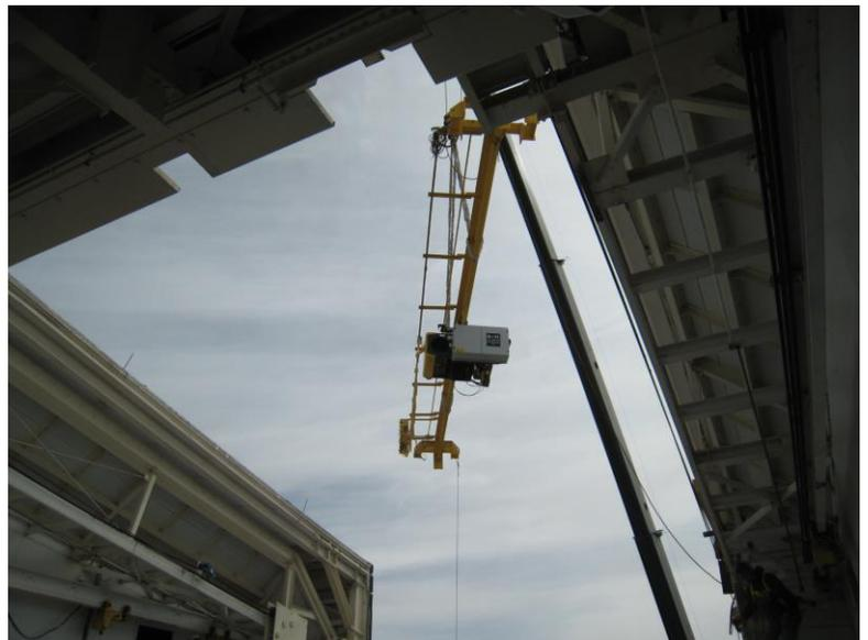
Moving the old 1978 bridge crane out of the chamber and the new 3-ton bridge crane into the chamber. For details, see page 18.
