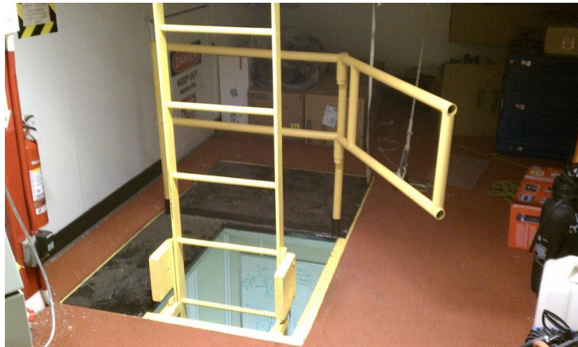
Figure 9. New guardrails installed in a 4 th floor loft area.
