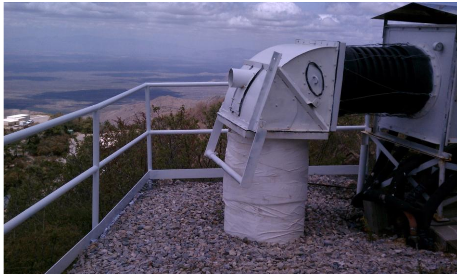
Figure 10. Guardrails installed around the shop heat exchanger.
