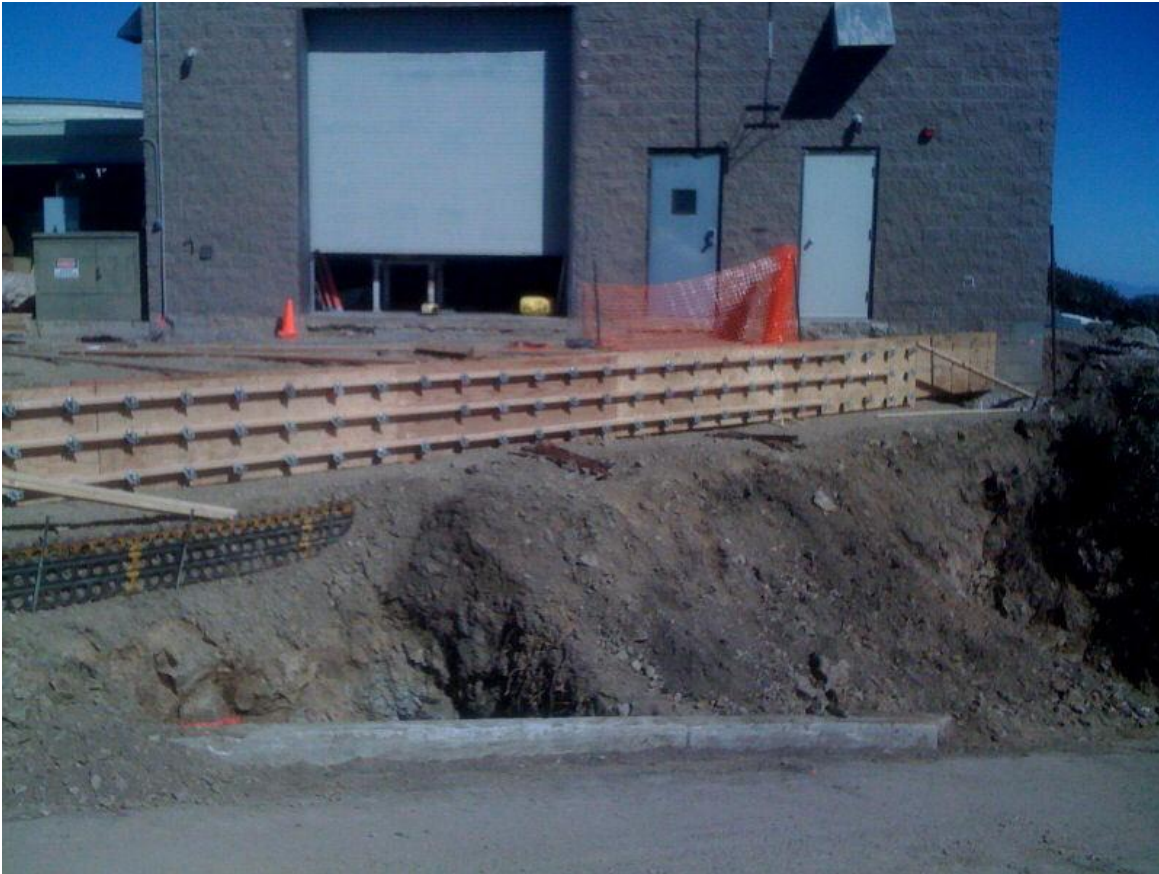
Fig. 8. Foundation preparations for instrument repair facility.
