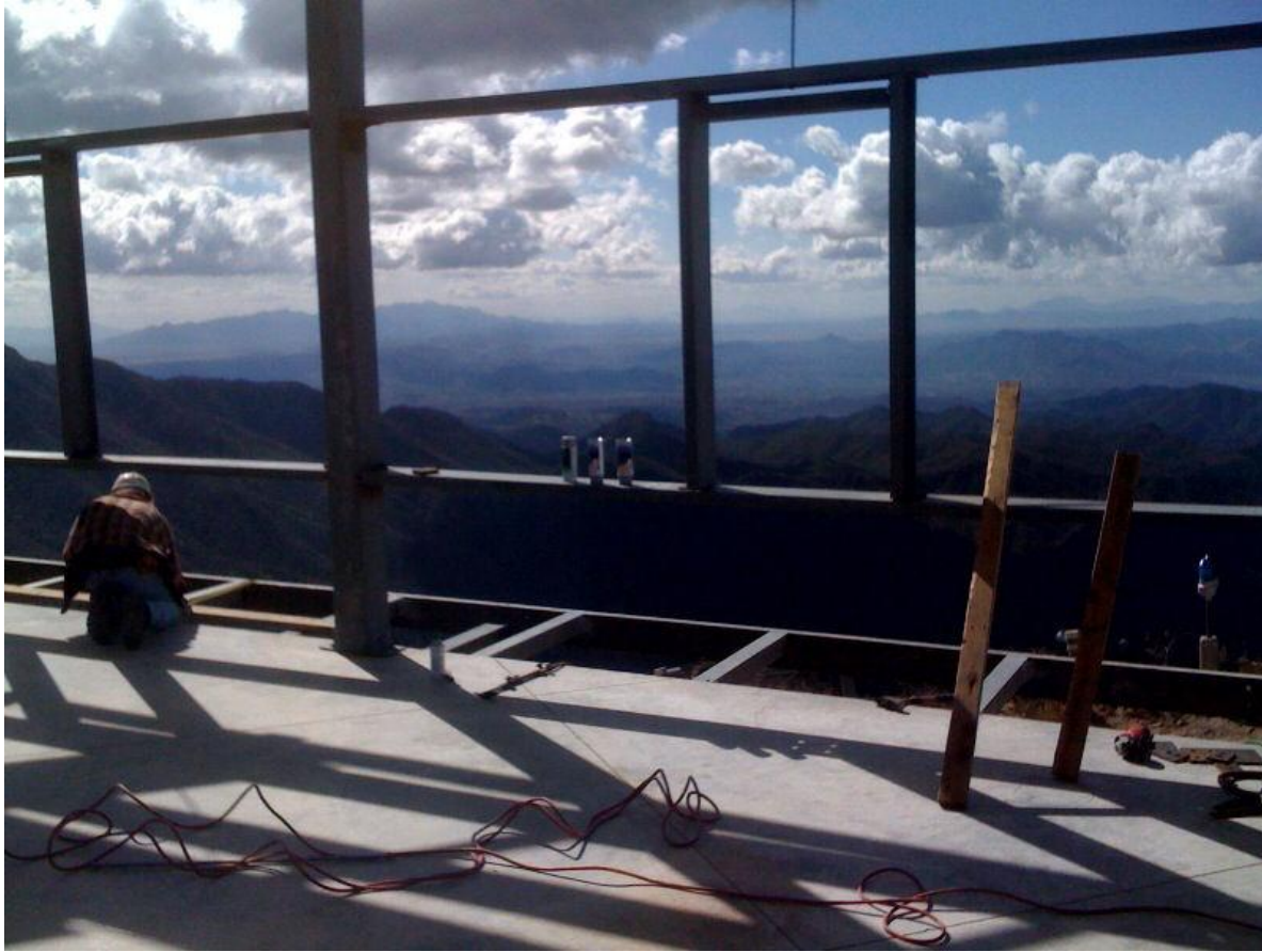
Fig. 10. New steel for the instrument repair facility.
