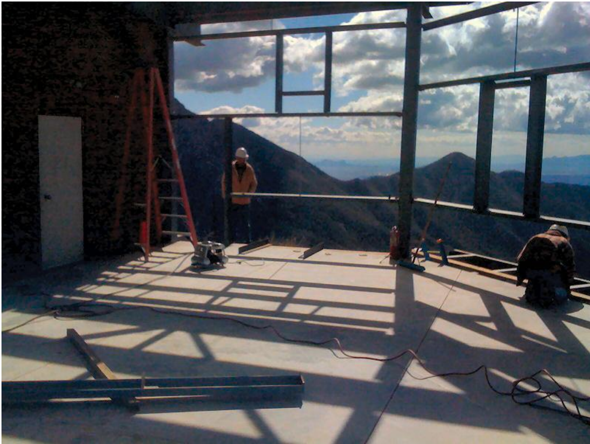
Construction of the new MMT Instrument Repair Facility
