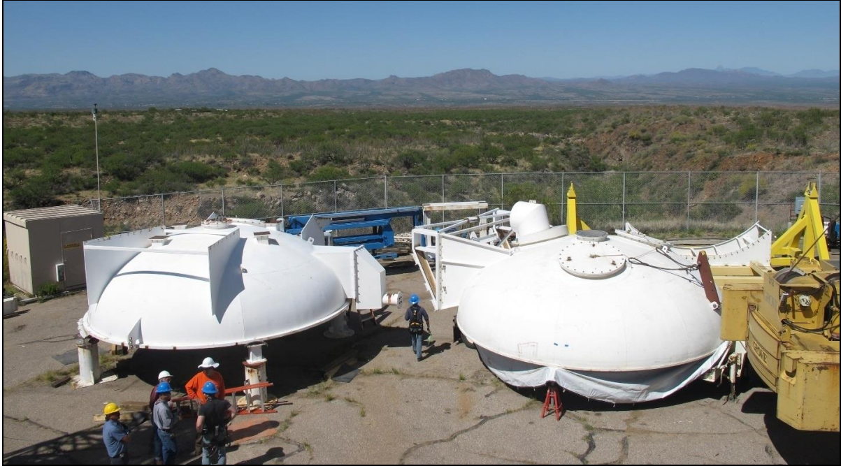
Figure 1. The rear bell jar and bell jar are shown before being placed on the tilt frame and cart.
