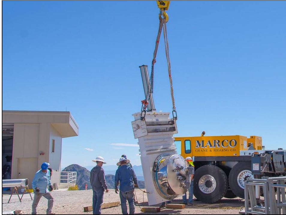
Figure 2. West cryopump being lowered onto blocks using newly fabricated handling fixtures.
