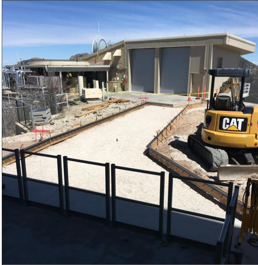
Figure 1. Support structures being prepared for a concrete pathway to be built between the IRF (shown) and the MMT main enclosure. The pathway will allow instruments to be easily moved between the two buildings.
